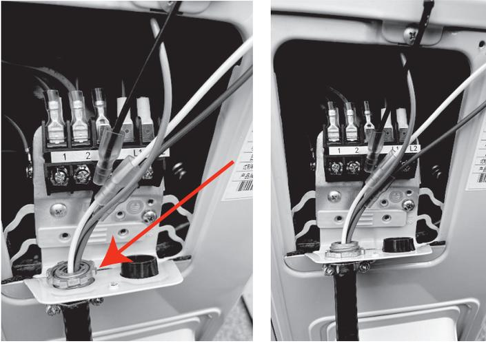
5. Then, you will connect the wires to the terminal block. Each wire should be numbered and correspond with a connection port on the terminal block. Match up each wire with the correct port, and firmly screw the u-lug of each wire to its corresponding terminal. Now, screw the ground wire into the bottom screw of the terminal block, as shown in the image below.
