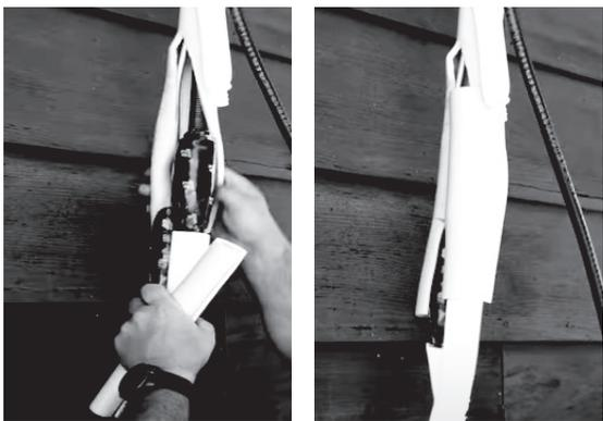
3. Now, starting at the outdoor condenser and working your way up to the wall hole, you will wrap the exposed line set and drain hose together tightly using the supplied Non-adhesive U.V. tape. The drain pipe will need to be at the bottom of the bundle (**Refer to Fig. 6.3 and the image below**). ***DO NOT*** wrap the end of the drain hose
