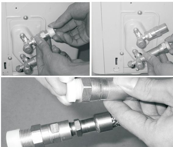
**NOTE:** Ensure the adapters attached to the outdoor valves have been tightened properly before attempting to connect the line set.
