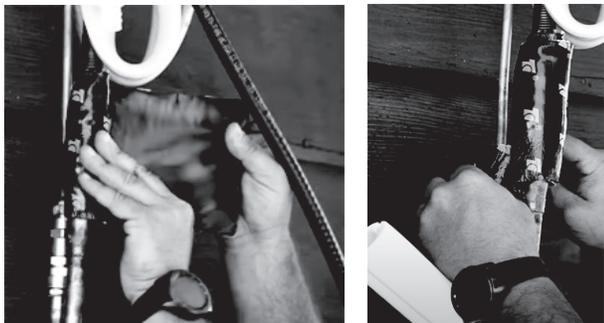
2. Now, place the supplied insulation material over the connectors and exposed refrigerant piping
